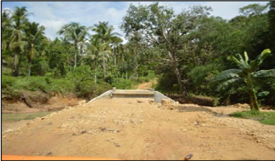
Figure 2.3-8 Road tracking proper in Leon B. Postigo
