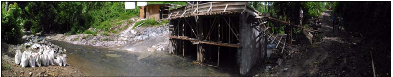
Figure 3.2.1-2 A Bridge Project Being Constructed
