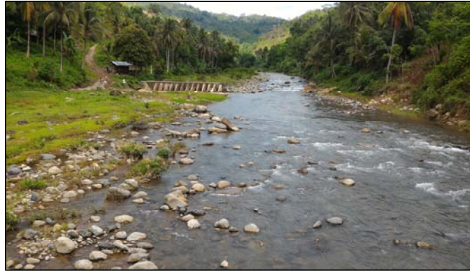
Figure 3.2.1-1 Unfinished Bridge Encountered During Road Tracking in Leon B. Postigo
